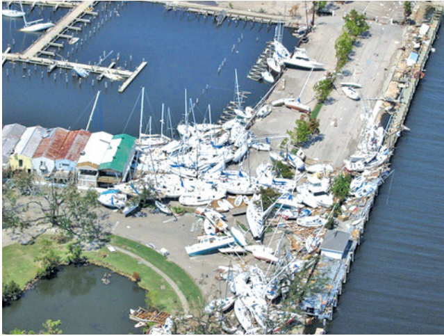
FIGURE 18: A marina damaged by Hurricane Katrina.
