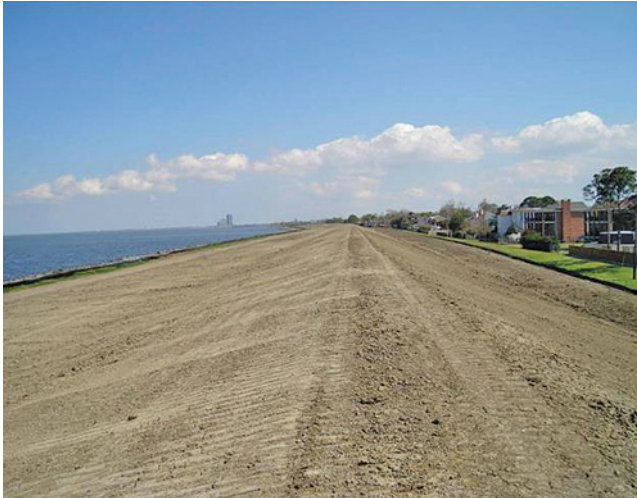
FIGURE 5: Raised levee near New Orleans.
