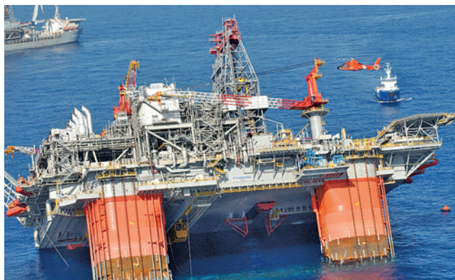
FIGURE 17: Hurricane damage to the Thunder Horse platform.
