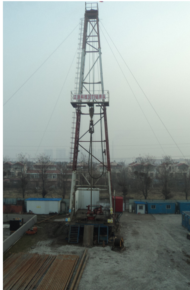
FIGURE 6: The drilling of the geothermal well at the Xiqing facility.
