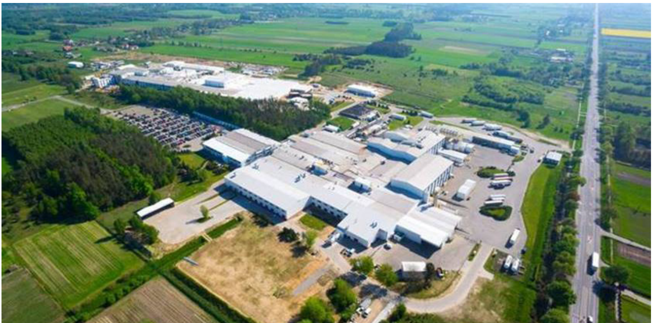
FIGURE 5: An aerial view of the Mars Production Campus, which includes the wastewater treatment expansion.
